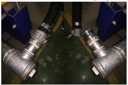
Open the 2" quarter turn valves on the end of the side pipes, if fitted.
